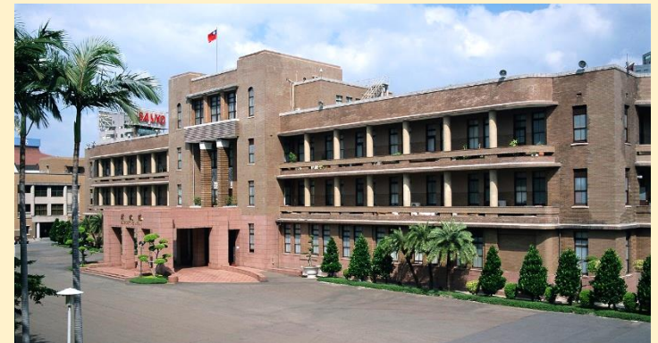
11 The front façade rises to a flat roof rather than a triangular pediment. At the main entranceway, a pair of columns with clean contours can be seen on each plane: square columns at ground level, ridged columns on the second level, and diamond-shaped columns on top.
